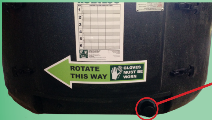
40mm Drain Plug on a Rota-Loo 650
