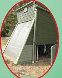
The Soltran Principal Clear sheeting is angled at 60 degrees with the largest surface preferably facing north. The rays of the sun heats up the cool air inside, the warm air is drawn into the Rota-Loo by the fan in the vent pipe. The front of the Soltran can also be used as the access door to the Rota-Loo room.
